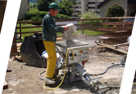
Injecting with bagged material for smaller jobs
