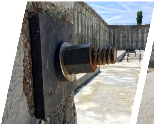
Sheet pile wall
