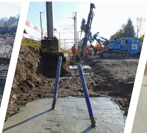
Foundation reinforcement
