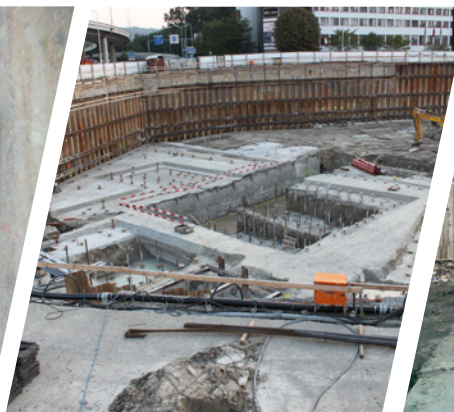
Retaining wall / sheet pile wall
