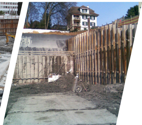
Pile / sheet pile wall
