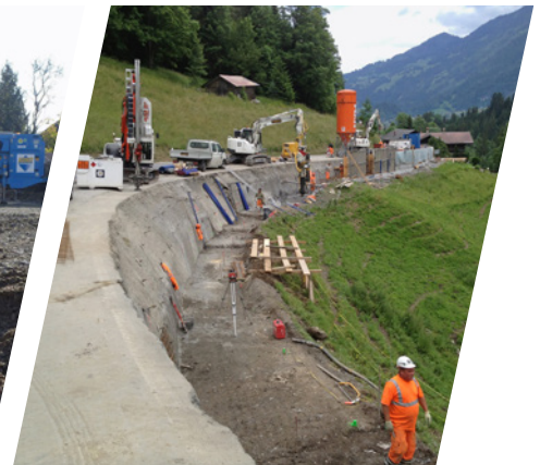
Embankment and road security
