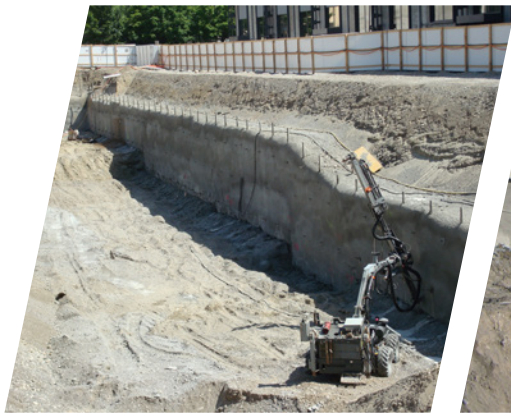
Rear anchored pile walls
