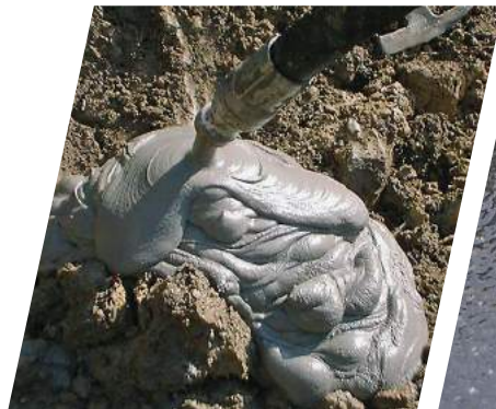
Filling with mortar, cement or KÜMIX®
