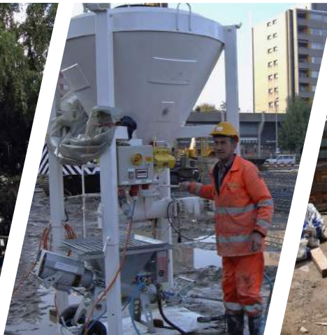
Injecting with bagged material or BIG BAG for smaller jobs
