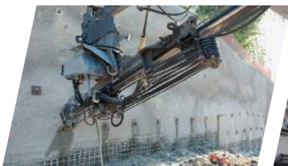
Self-drilling anchor
