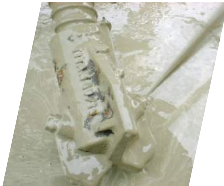
Jet grouting with KÜMIX® (40–150 bar)
