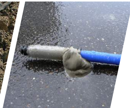
Re-injection with cement or KÜMIX®
