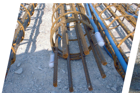
Attachment of K Injection pipes
