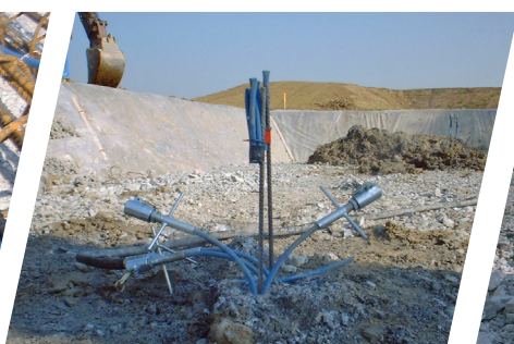
K Re-injection connections rupture pressure approx. 15–65 bar after 24 hours
