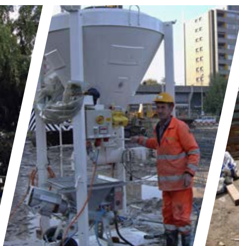
Injecting with bagged material or BIG BAG for smaller jobs
