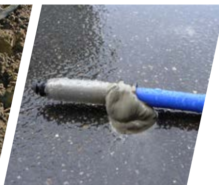
Re-injection with cement or KÜMIX®
