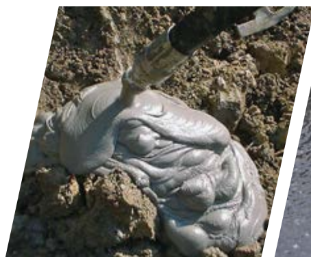
Filling with mortar, cement or KÜMIX®
