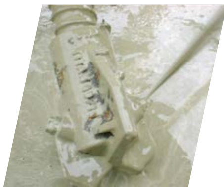
Jet grouting with KÜMIX® (40–150 bar)
