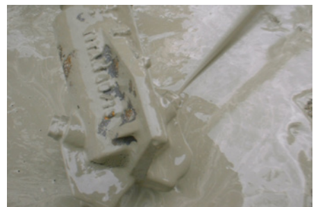
Jetting 400 bar/ KSB Jet
